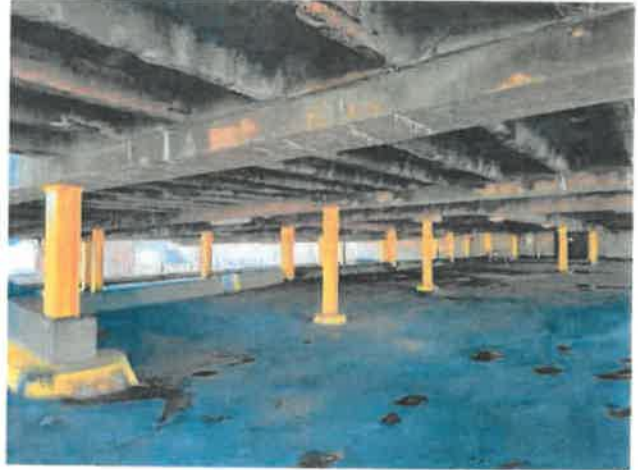
Photo 10 - Pan-Joist Deterioration
