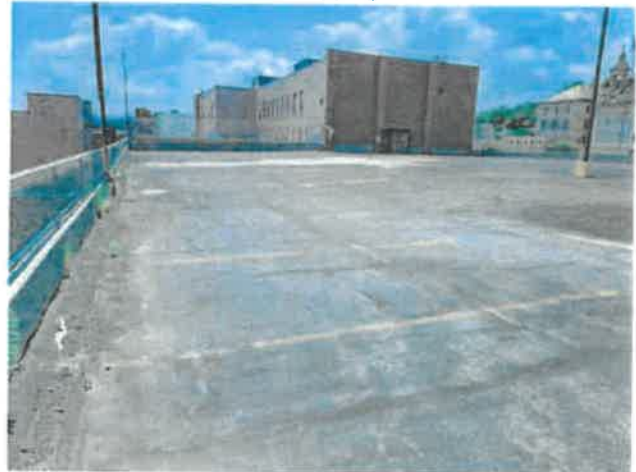
Photo 12 – Top level traffic topping
