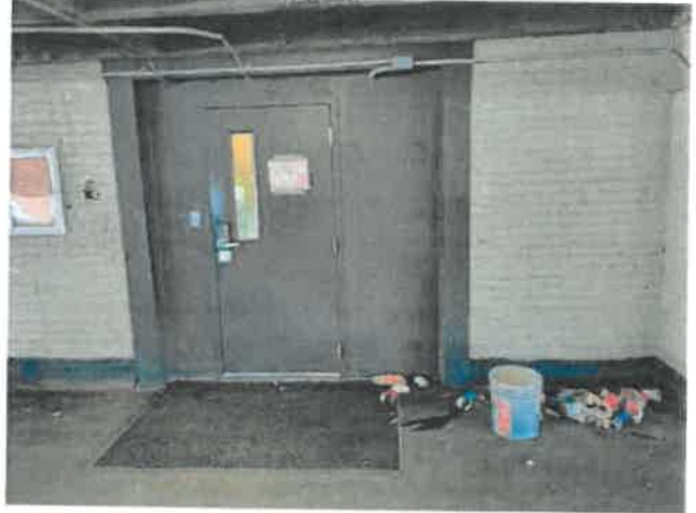
Photo 18 – Typical door to adjacent occupied space
