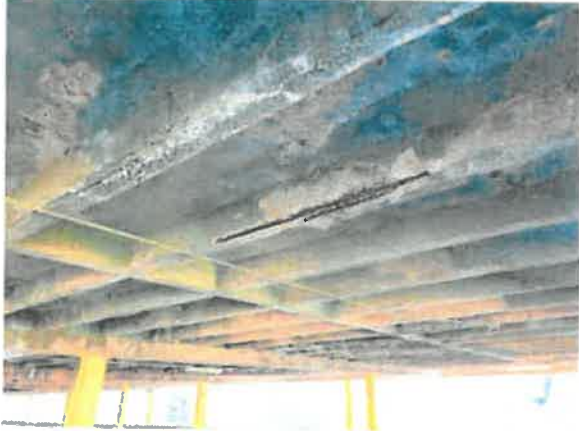
Photo 9 – Pan-Joist Deterioration
