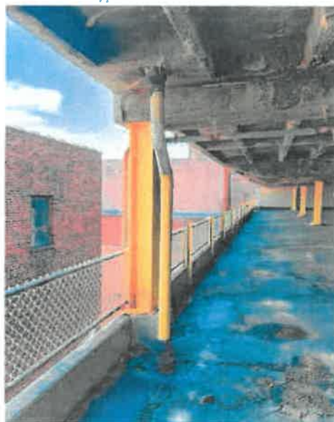
Photo 16 – Typical column and drain
