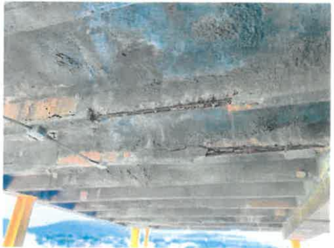
Photo 8 – Pan-Joist Deterioration
