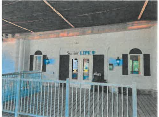
Photo 22 – Level 3 door to occupied space
