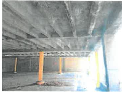
Photo 6 – Pan-Joist Deterioration
