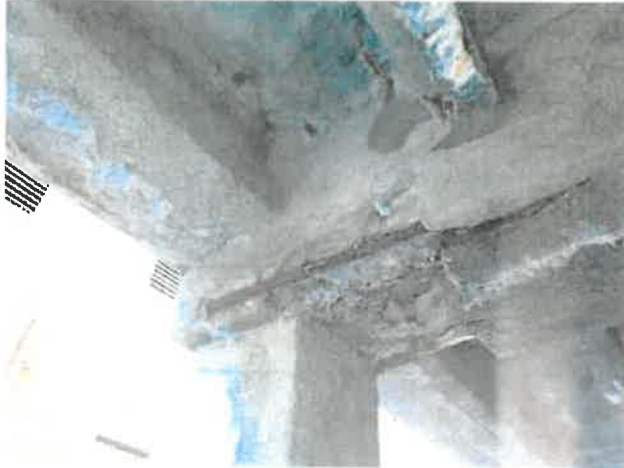
Photo 5 – Girder deterioration
