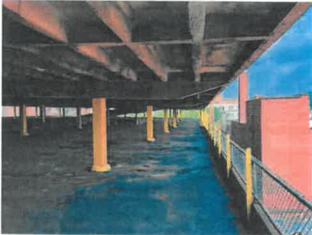
Photo 7 – Pan-Joist Deterioration
