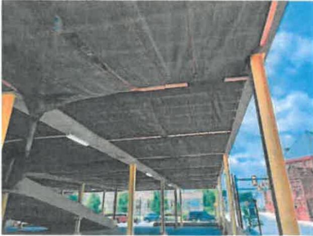
Photo 21 – Netting under Level 4
