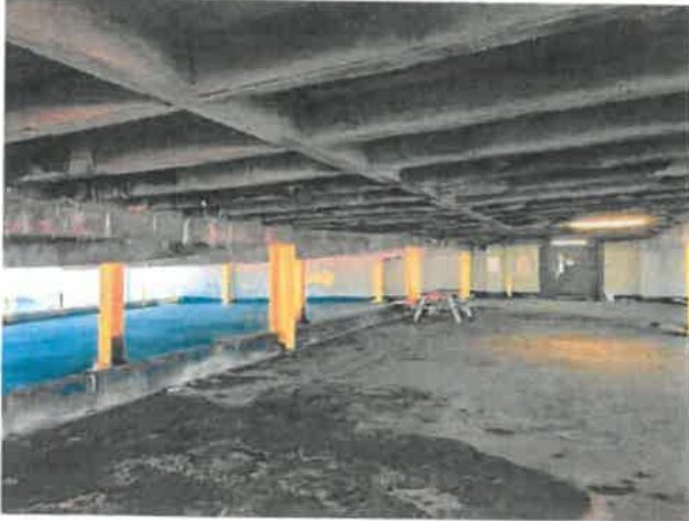
Photo 11 – Pan-Joist Deterioration
