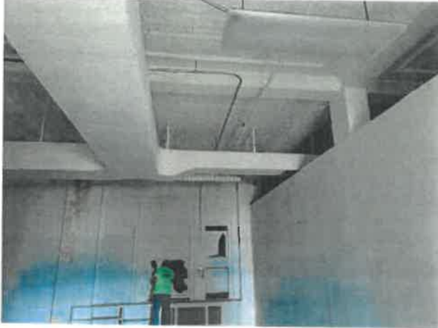
Photo 25 – Interior finished space
